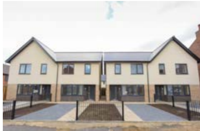
Some of the completed homes
