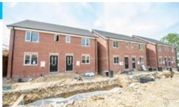
Some of the new houses being built
