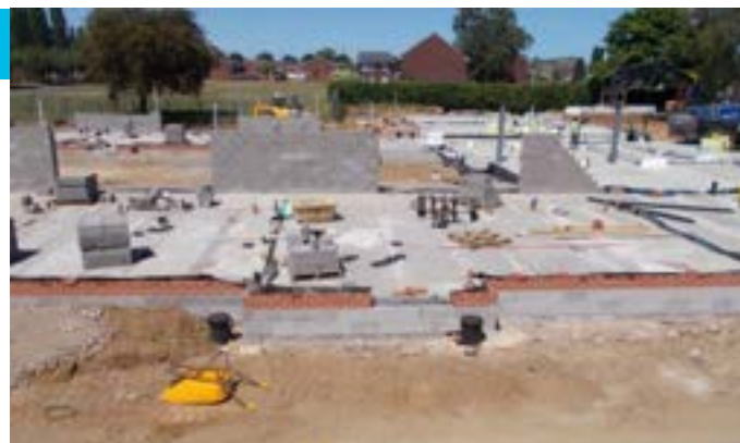
Building work well underway
